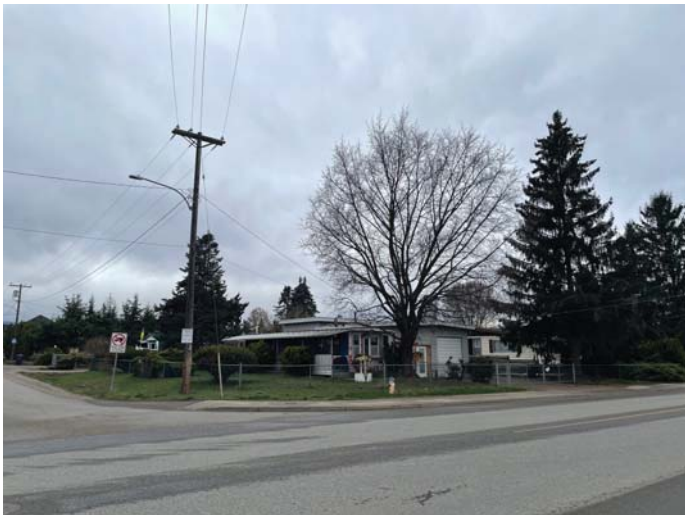
EXISTING HOUSE FROM MCCURDY RD LOOKING WEST
