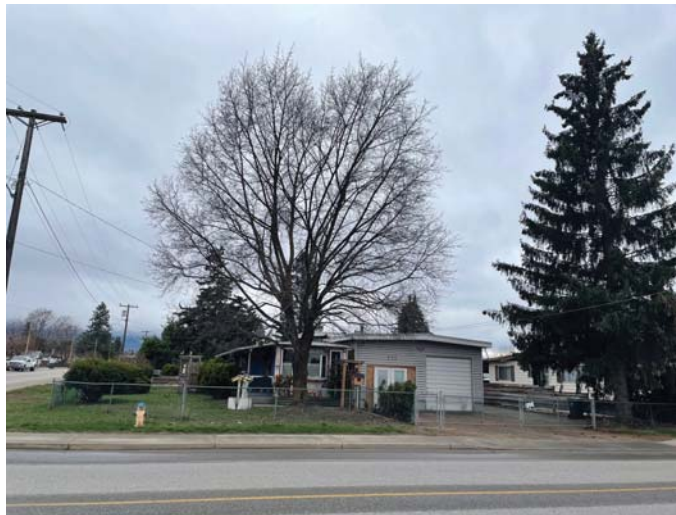
EXISTING HOUSE FROM MCCURDY RD LOOKING WEST
